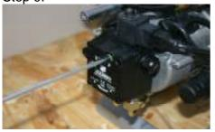
After setting the measurement data and burner output, switch off burner, screw out manometer, screw in plug and put burner into service.
