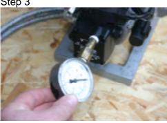
Burner oil pump: Screw out plug on the pump lid using the Allen key provided (P) and screw in manometer for purposes of monitoring and alteration of pressure settings changes.
