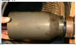
Open boiler door, pull off flame tube with bayonet mount and clean it.
