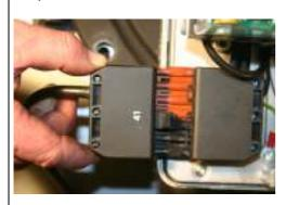
Remove electrical connection from boiler at burner Euro socket and switch off boiler system.
