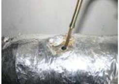
**Upon burner startup** – Insert measuring probe from the emissions device into the measuring opening on the exhaust gas tube and observe exhaust gas values.
