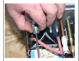
As required, open or close air valve for combustion air in relation to measured data.
