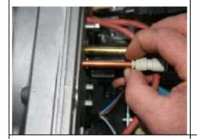
Pull ignition cable off of the ignition electrodes.
