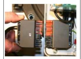
Connect electrical power line from boiler to Euro plug on C1 burner.
